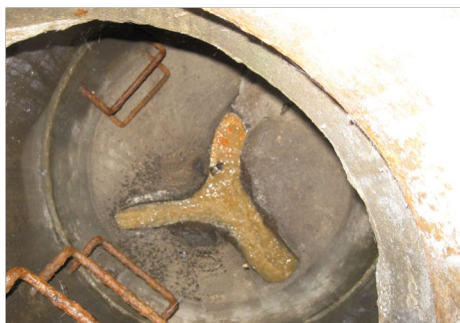
Grease clog in sewer.
